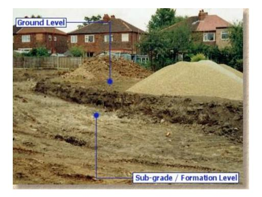
An area between ground level and subgrade / formation level need to scrap off due to the instability of the soil. This EARTHWORK procedure consist of clearing, grubbing, cut and fill that includes excavations of soils.
