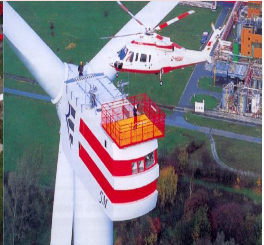
Use Of Helicopters For Lifting
