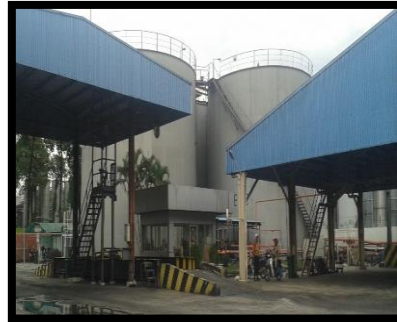
CPO STORAGE TANK
